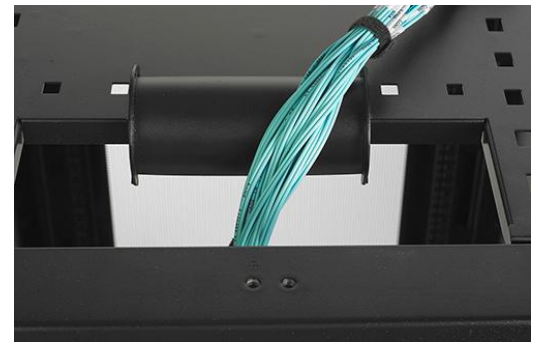
Installed on rear roof hole of AR3100
